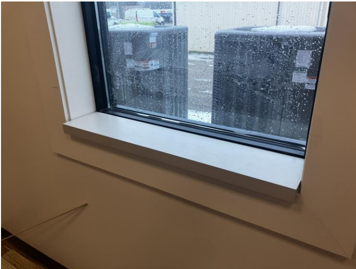
13. Windowsill and SF-3 in Staff 116
