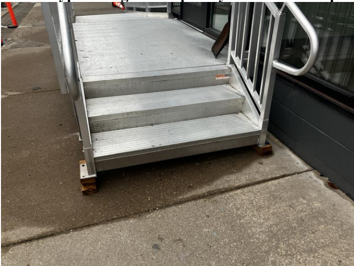
17. Temporary Stair at Sidewalk
