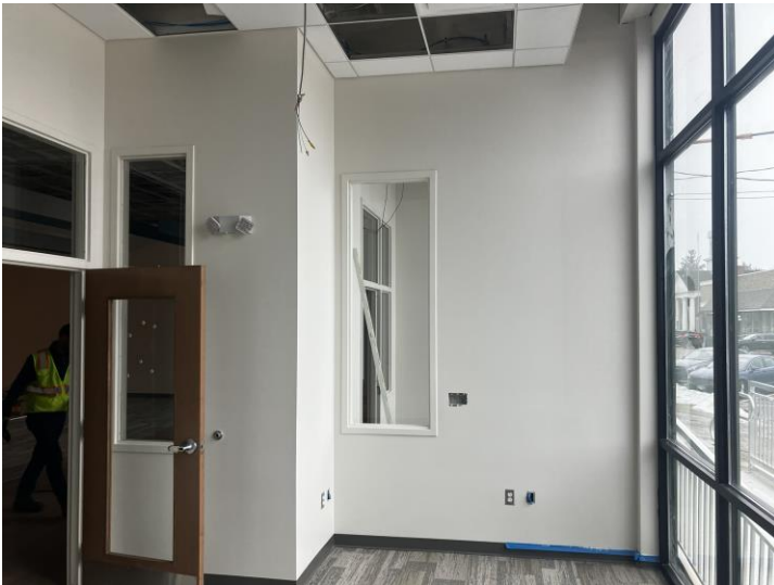
3. Work Room 101, Looking West
