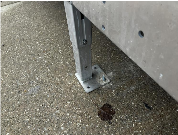
16. Typical Leg at Temporary Stair and Ramp
